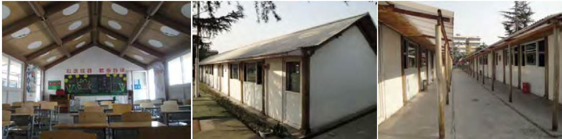
Figure 7 – 9 From left to right: Inside the classroom; Outside the classroom; The courtyard space between the classrooms
