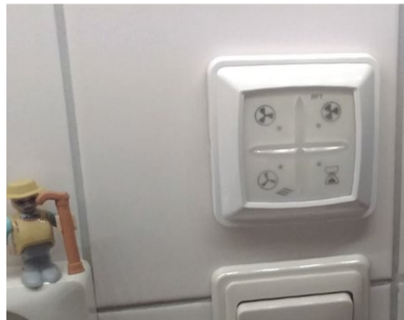
Figure 7 Selecting the function suitable for the situation: no indication of the setting the control is currently on.
