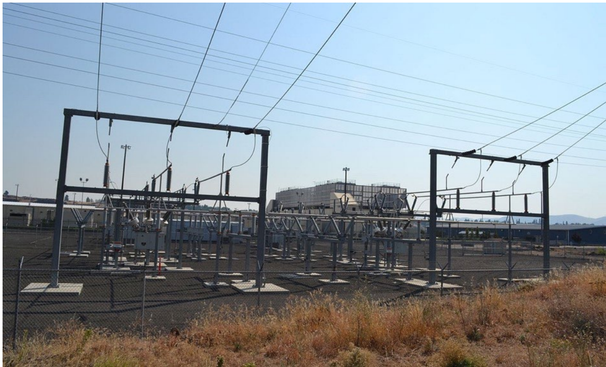
Figure 4 The exterior of Google's data centre – 'The Dalles' – in Oregon, USA (Visitor 7, 2011, https://creativecommons.org/licenses/by-sa/3.0/deed.en ).
