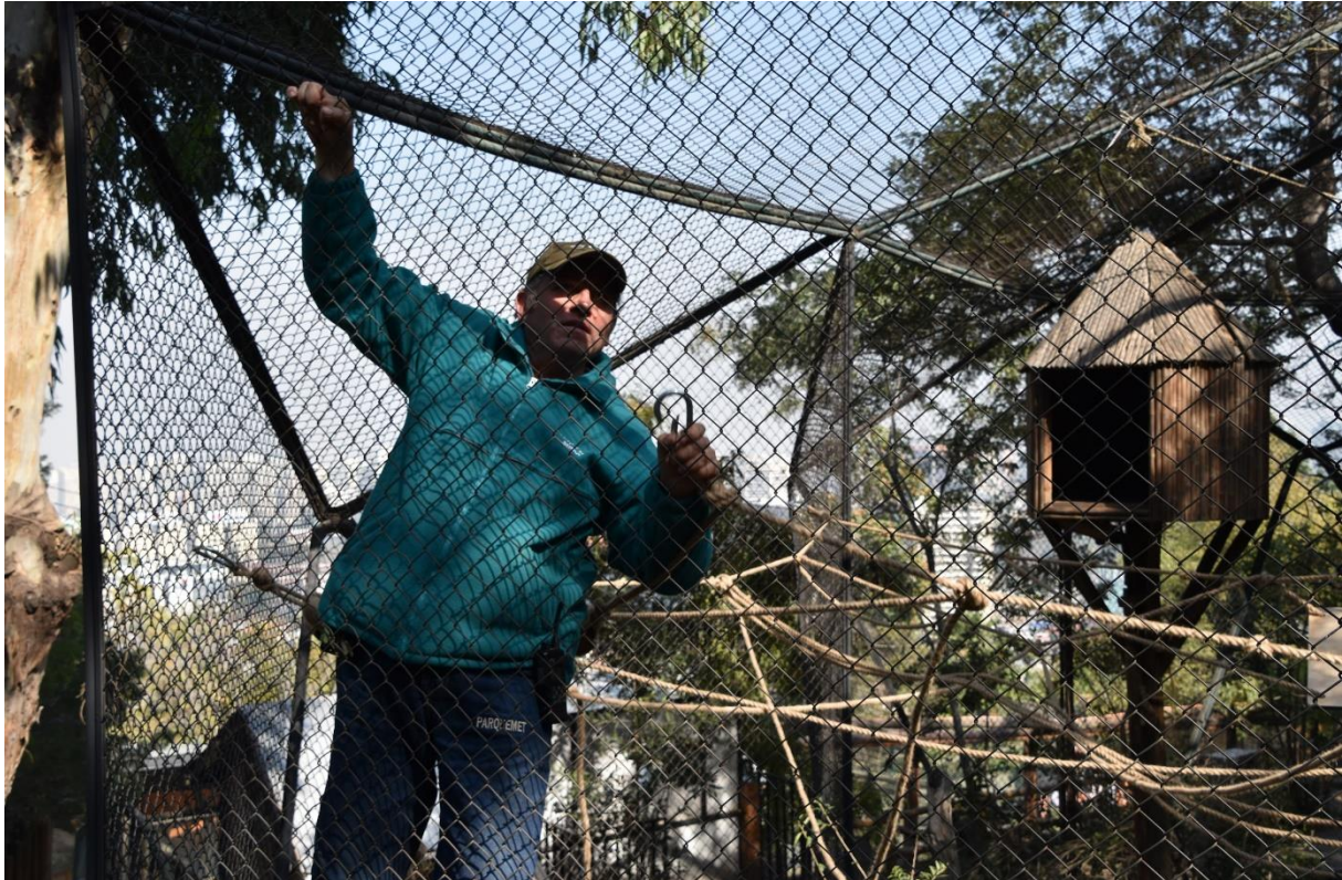
Figure 3: General view of the installation of the second prototype (Gibonas, 2016).
